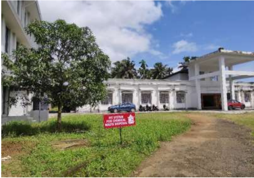
Figure 5 LABORATORY WASTE COLLECTION PIT
